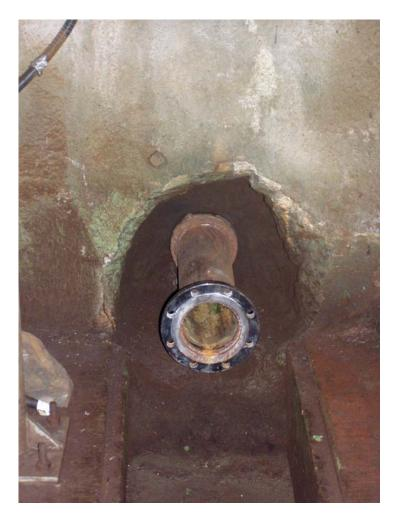
View of new slop line from lower tunnel before installation of 6" valve.
