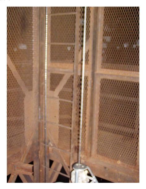
Area where elevator cage was removed at the platform level – note the relocated ladder.
