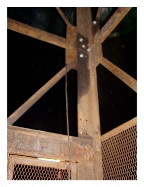
Typical area of replaced fasteners - note plug weld repair of flame cut holes.
