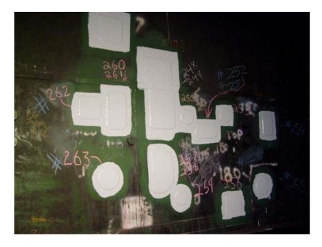
Typical patch plate repairs (note the Dunkin & Bush assigned flaw numbers)
