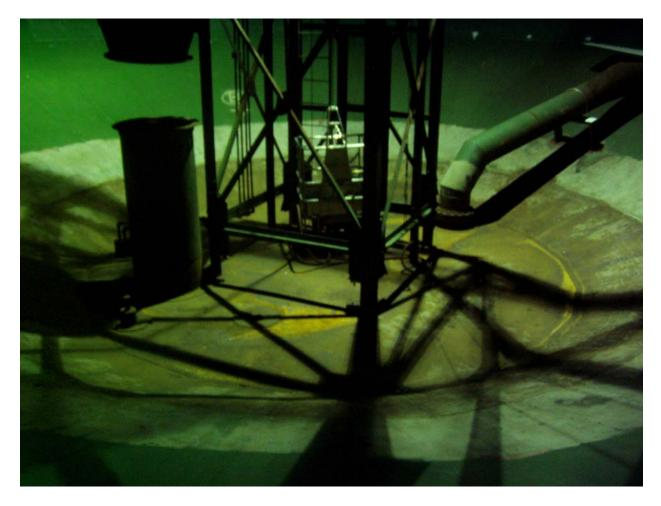
View of tank 15 bottom area where gauging equipment and attachments were removed
