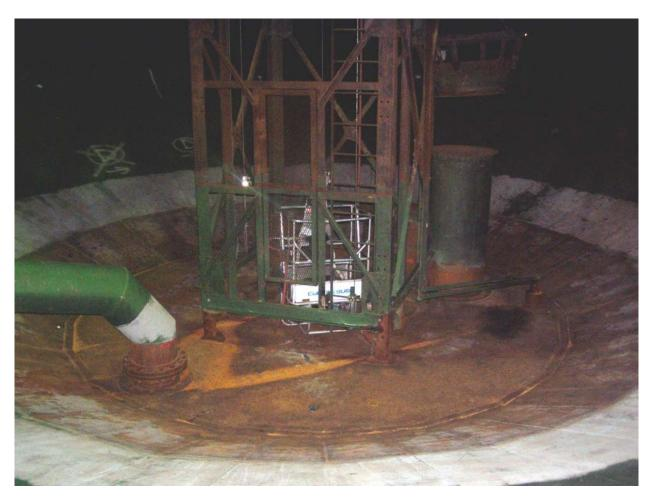
Tank 15 bottom after anchors and clips were removed. Also note where the elevator landing platform and steps were removed from the facing side of the tower structure.
