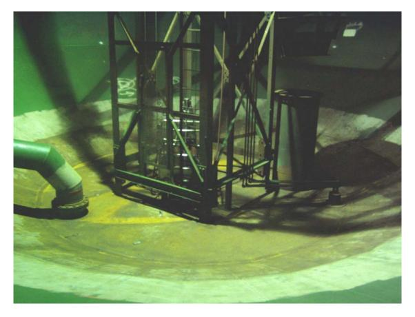
View of tank 15 bottom area where the elevator platform and steps were removed.
