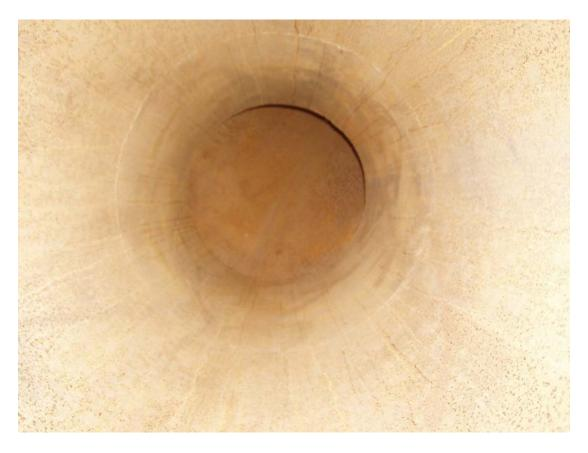
View looking down the 32" line from inside tank 15. Note the circumferential weld before the bend. This is weld repair "A" identified in the Weston Solutions sketch.
