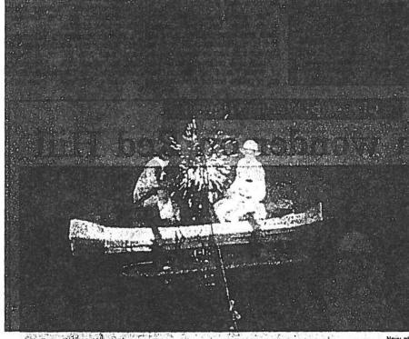
Workers in a cance weld shut a leak in the wall of a water-flooded fuel tank. the sea tomas int Nevy photo
