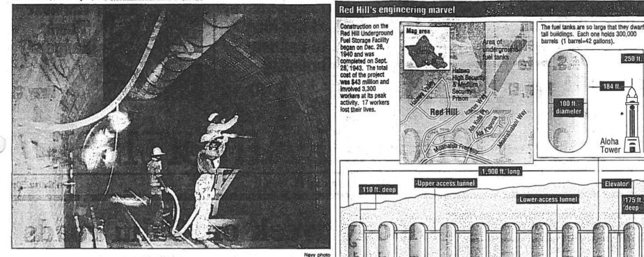
In this historic view, workers spray concrete onto the walls of a tunnel connecting the fuel storage tanks beneath Red Hill.
