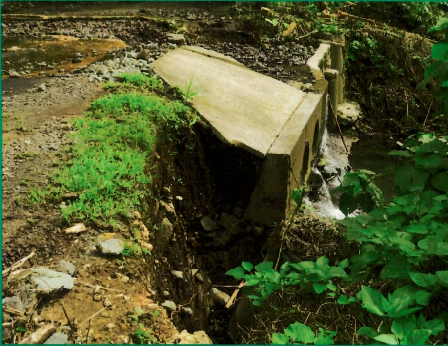
Road and culvert partially washed away at stream crossing
