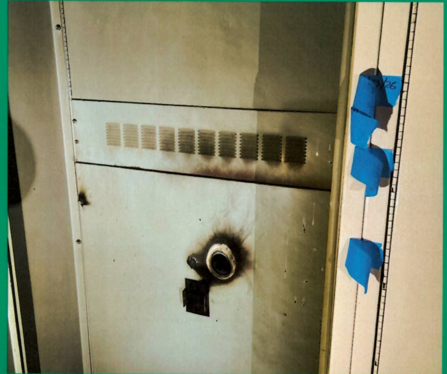
Indications of an electrical fault within the control building motor control switchboard were observed.
