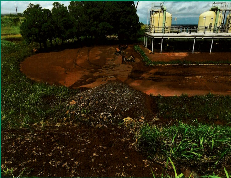
Land Slide – landslide that coated the GAC treatment area with mud and dirt
