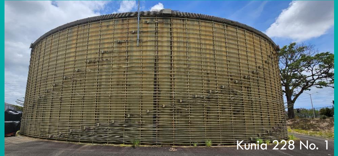
External Post-Tensioned Tank
