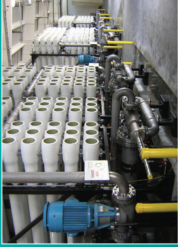
Typical RO treatment facility – Kalaeloa Desalco
