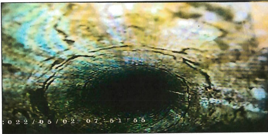
Top of Well (galvanized pipe inside outer iron pipe)
