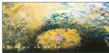
Algae and Sediment in Bottom of Well
