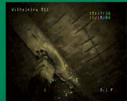
Significant spalling and exposed reinforcing in roof slab support beams. Deterioration is severe.
