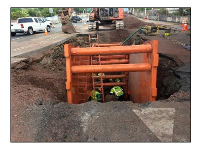
Once the trench box was in place, hand excavation got underway as the only feasible digging option.
