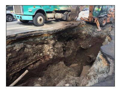
As is shown here, absent the trench box installation, the sides of the hole would be subject to caving in.
