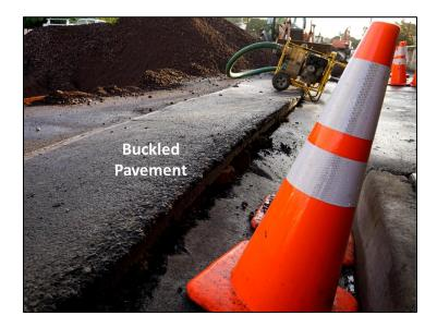
The force of the water had buckled the pavement, between 6 inches and more than a foot.
