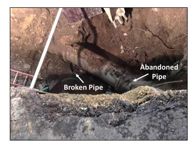
An abandoned pipe was found crossing the broken pipe at a higher elevation. This limited access to the broken pipe.
