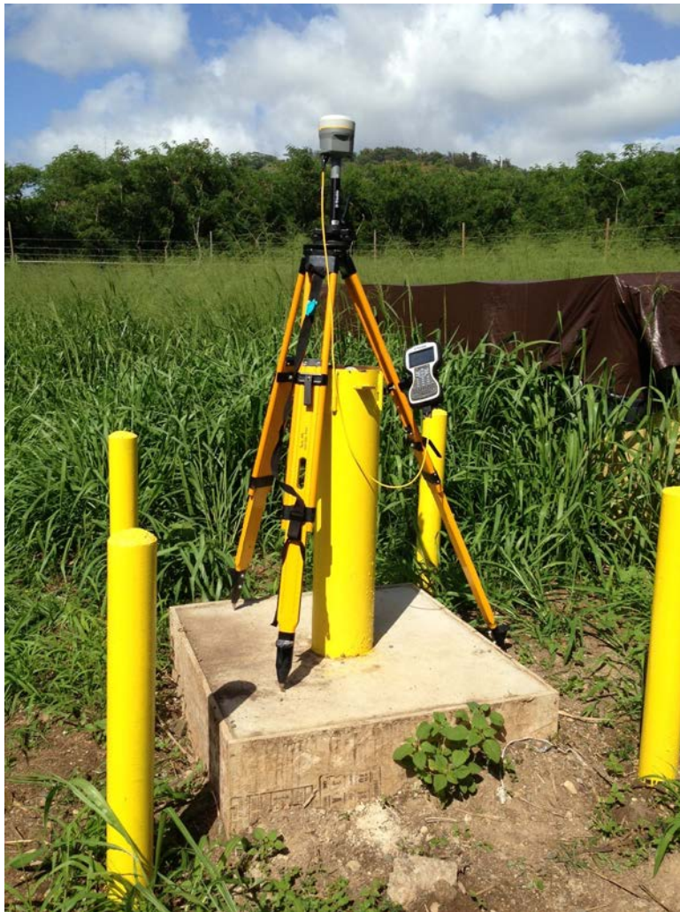
Figure 1. New Monitoring Well
