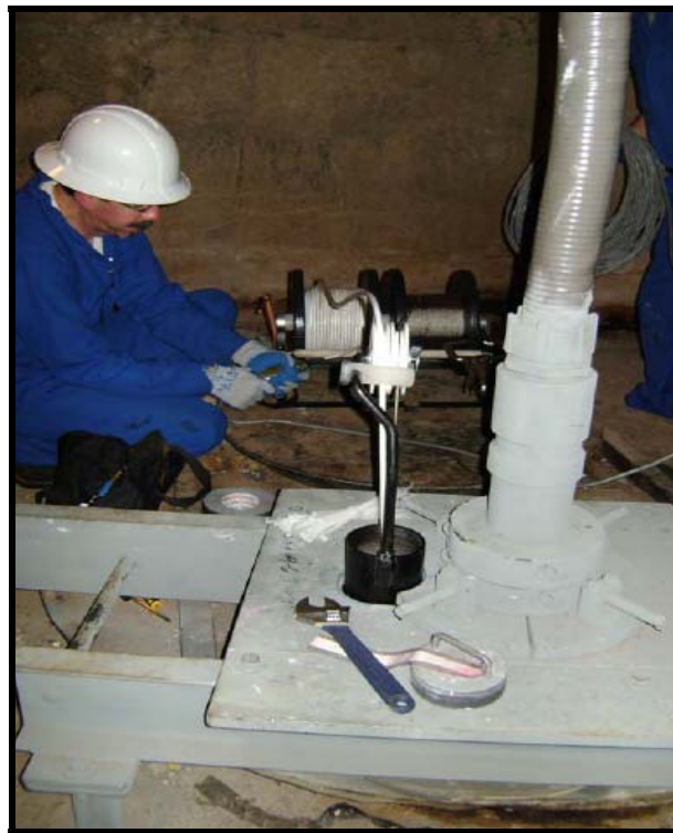
Figure 1-3: Typical Tank Top Access
