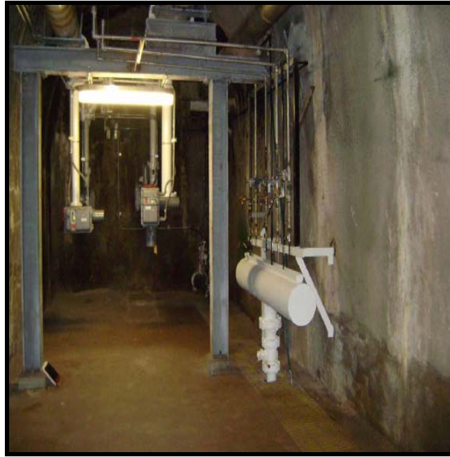
Figure 1-2: Typical Tank Bottom Access
