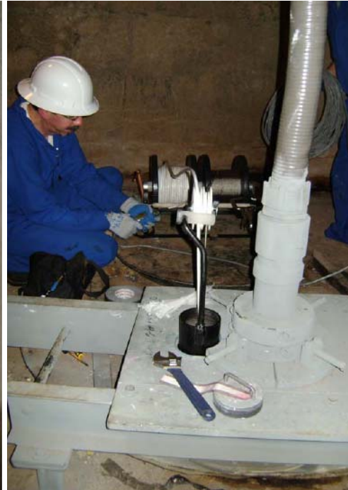
Figure 3: Typical Tank Top Access
