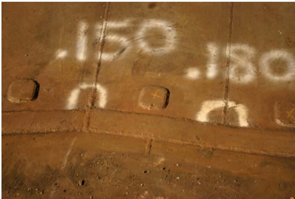
Photograph 12 – Lower dome and the bottom of the tank. Note the flaws marked at the intersection of the lower dome plates and bottom plates.
