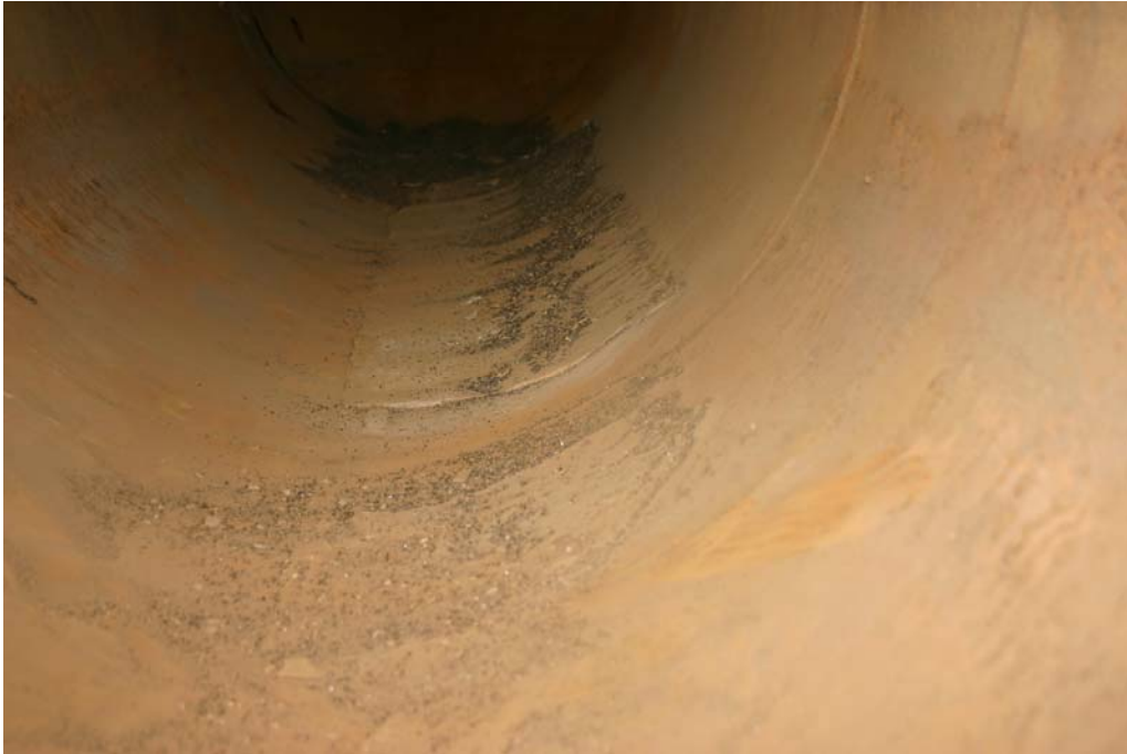
Photograph 9 – Poorly adhering thick-film coating inside the 32” nozzle at about the 35’ to 45’ stations
