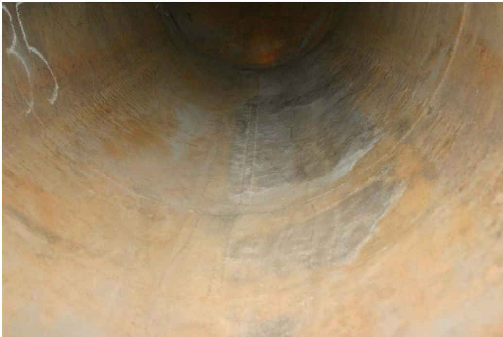
Photograph 10 – The same section of piping after the poorly adhering thick-film coating was removed. UT measurements indicate that the corrosion in this area of the pipe is not extensive and the coating appears unnecessary and somewhat ineffective when the surface preparation is not completed correctly.
