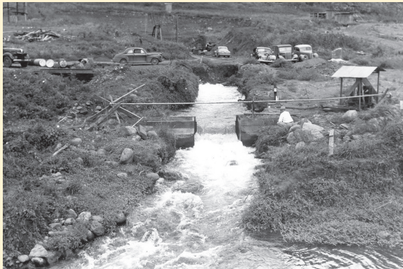
Water had to be pumped out to keep water levels low enough to work. It is estimated that 20 million gallons per day was pumped during construction in the 1940s, enough to fill 30 Olympic-sized swimming pools.
