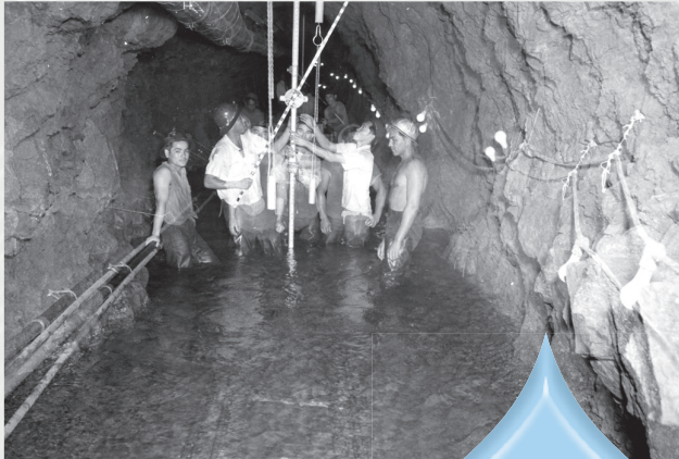
Construction workers excavated the 10-foot high tunnel while waist-deep in water.
