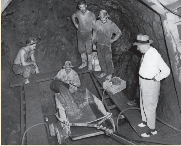
Miners bailing out water that seeped into Hālawā Shaft. The Board of Water Supply's first Manager and Chief Engineer, Fred Ohrt, is at right. September 11, 1942.
