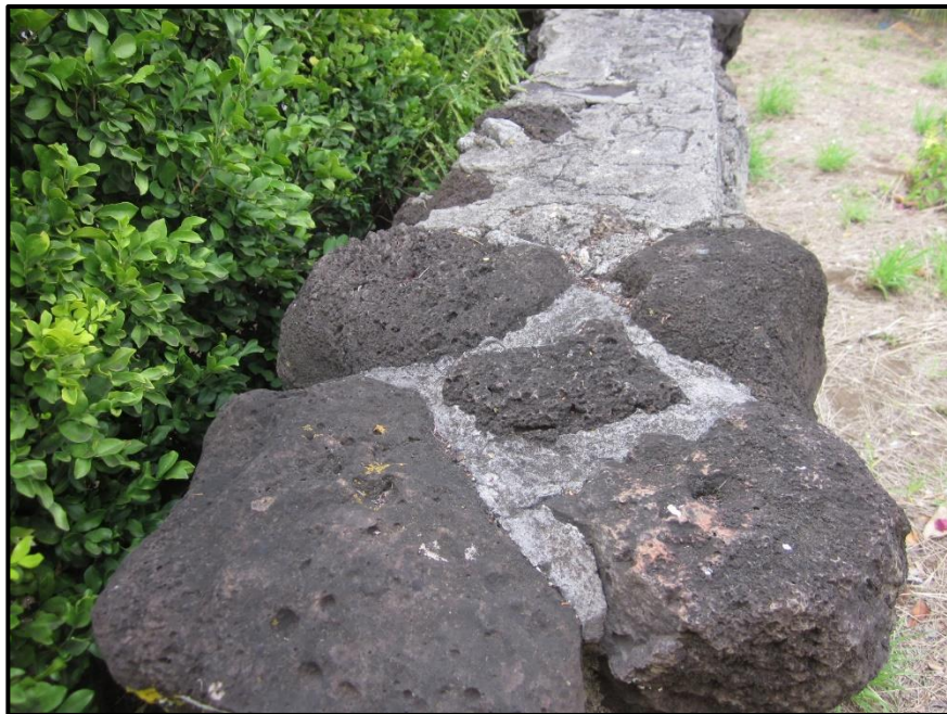
Figure 41. Photographs of the Top of Feature 33 Retaining Wall and Feature 33.1 Entry Pier. Top: North End of Feature 33 Showing Grooved Mortar, View to East. Bottom: Feature 33.1 Top of North Entry Pier Showing Mortar and Concrete Boulder Cap, View to South.
