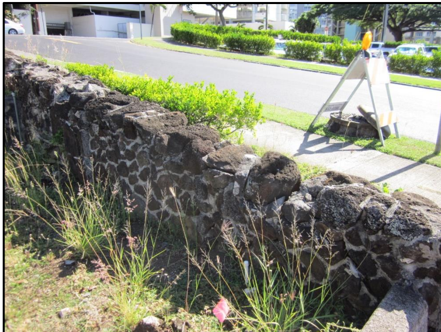
Figure 46. Photographs of Site T-1, Feature 34, Retaining Wall. Top: Feature 34, View to West. Bottom: Feature 34 Showing Top of Wall Capped with Boulders. View to East.
