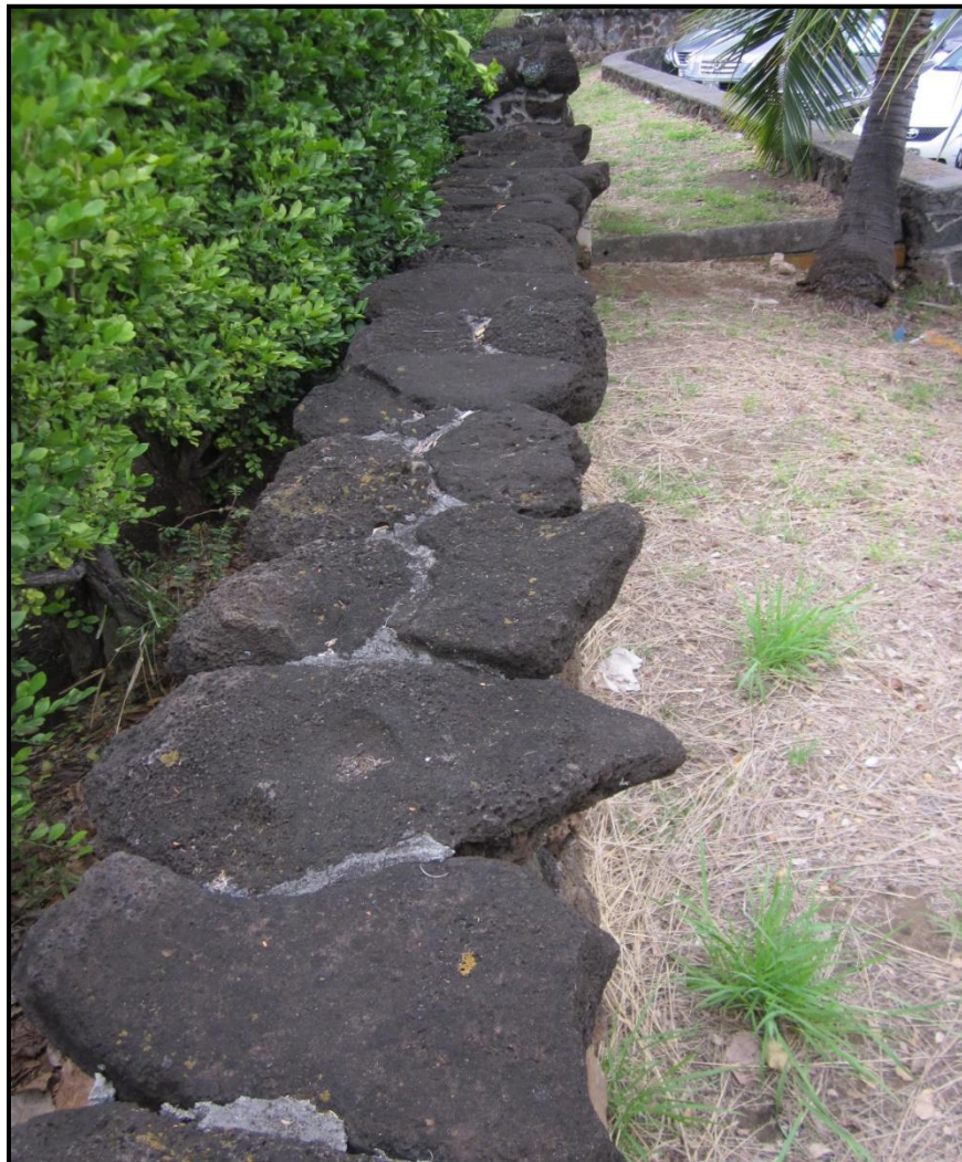
Figure 39. Photograph of Site T-1, Feature 33, Top of Retaining Wall Showing Boulder Cap, View to South.
