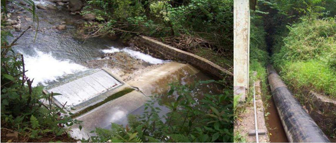
**Figure 1.7 Punalu’u Stream Diversion and Piped Ditch**
