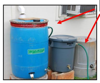
These rain barrels have an overflow near the top. The hose for the overflow can either be directed towards your yard or into another barrel.
