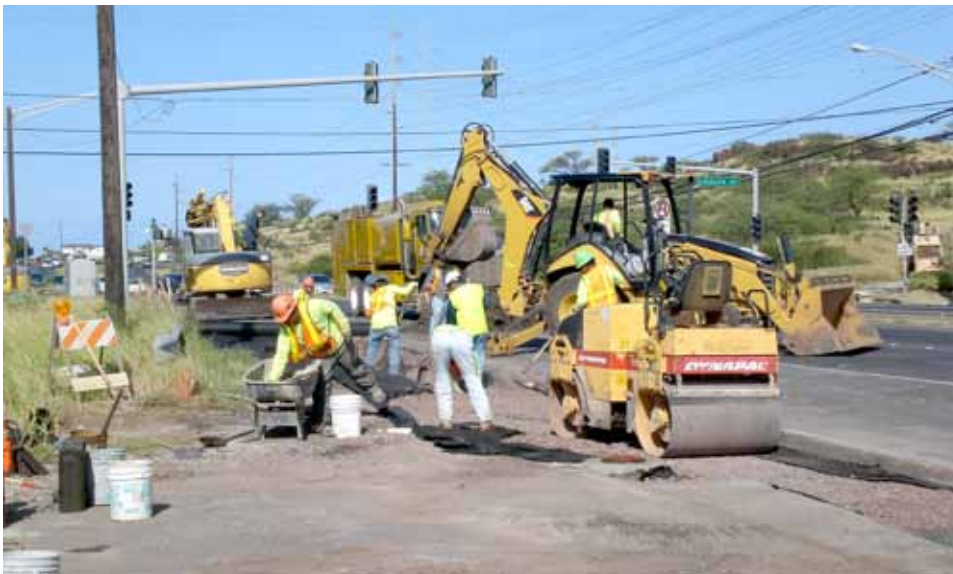
Water System Improvements. The BWS completed the water system improvement project along Farrington Highway in Nanakuli. The new 24-inch transmission line provides approximately 60-percent of the drinking water into the Leeward Coast.
