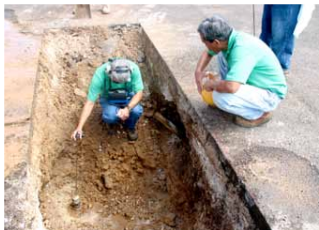
Leak Detection Program. The BWS Leak Detection Team proactively looks for and identifies leaks in the BWS system. The data collected is used to schedule planned repairs to the water system.
