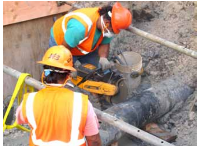
Water Main Breaks. BWS Field Operations crews respond to emergency water main breaks to minimize water loss and restore water service as soon as possible.
