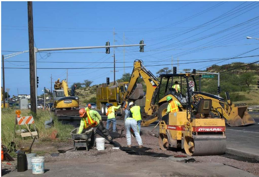
***Water System Improvements. The BWS completed the water system improvement project along Farrington Highway in Nanakuli. The new 24-inch transmission line provides approximately 60-percent of the drinking water into the Leeward Coast.***
