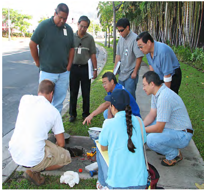
Corrosion control testing BWS engineering staff learn how to collect information from corrosion control equipment to test and determine the most effective methods available to extend pipeline life expectancies.
