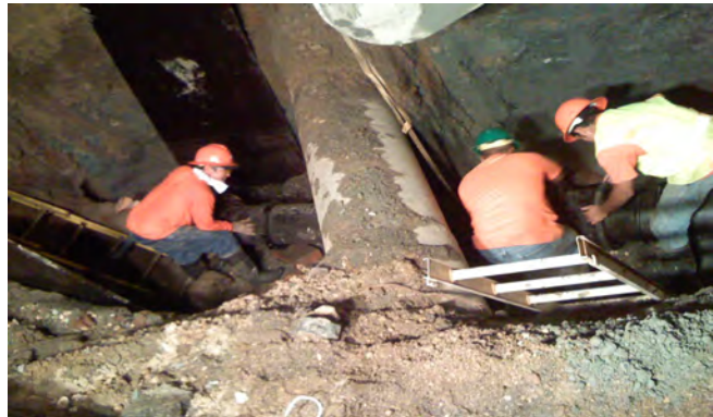
September 2007 Keolu Drive main break. BWS crews often work in muddy trenches under incredibly challenging conditions, day and night, to quickly restore water service to customers.
