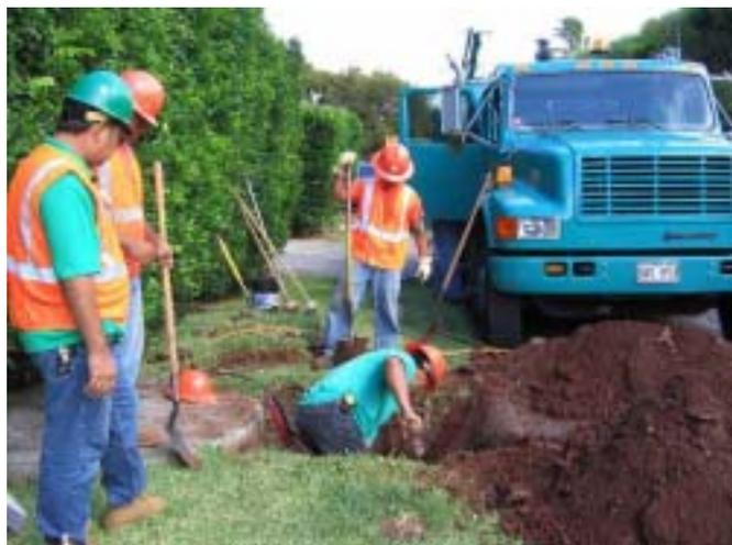
*Internal Conservation. Surveying and checking the more than 2,000 miles of underground water lines and mains for leaks and other problems have resulted in major water savings in unaccounted-for water use and loss due to leaks.*
