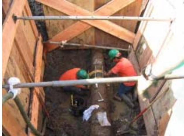
**Main Break Repairs.** BWS crews need to excavate and expose the pipe before leaks or breaks in the water main can be repaired. It continues to be a top priority with the BWS and its employees to ensure the prompt repair of all broken pipes and to restore water service to affected customers.
