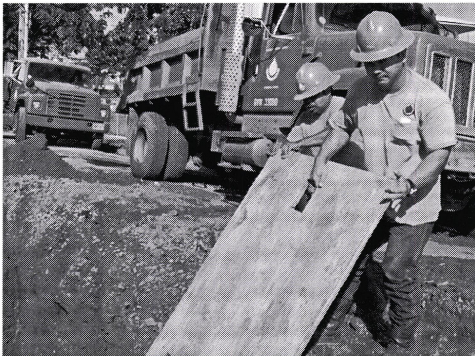
Men at work. Field crews in the Multi-Skilled Worker pilot program undergo extensive training to learn each other's job skills – such as pipefitting, carpentry, masonry, and operating construction equipment – to become proficient in each trade. The goal of the program is to streamline operations, improve productivity and improve customer service.
