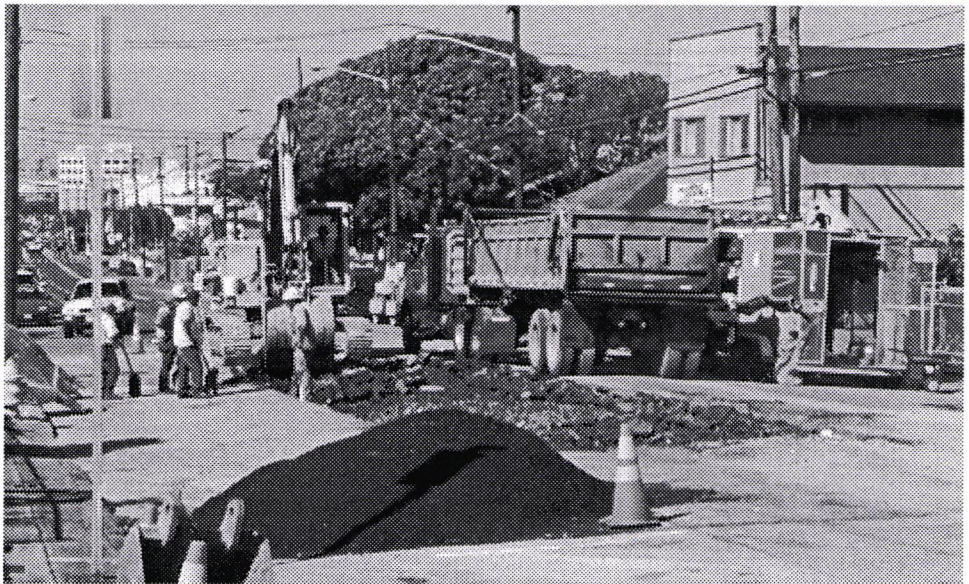
Emergency repair. This past fiscal year, the BWS responded to 400 main breaks such as this one on Liliha Street.
