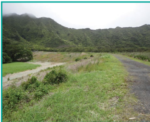
Do Not Walk on private roadway along the top of Nuuanu dam & reservoir.
