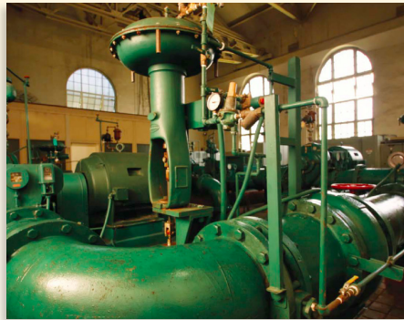
Pumps at the BWS Beretania Pump Station extract water from underground aquifers and move it to reservoirs in the area.
