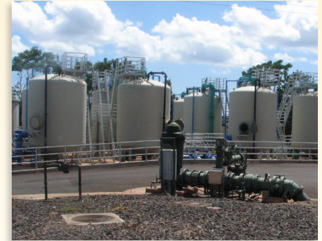
Granular activated carbon treatment facilities remove legacy agricultural contaminants from the drinking water supply in Central O'ahu and 'Ewa-Waipahu.
