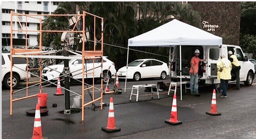
Advanced pipeline condition assessment requires traffic control, excavation, construction of a vault, tapping into water-filled pressurized pipe, and installation of a valve. The testing team tracks a probe inserted into the pipeline, propelled by the moving flow of water, up to a distance of ½ mile.
