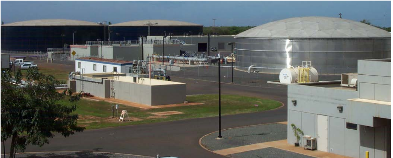
Honouliuli Water Recycling Facility. The facility continues to offset potable water demand by producing recycled water as an alternative for irrigation and industrial purposes
