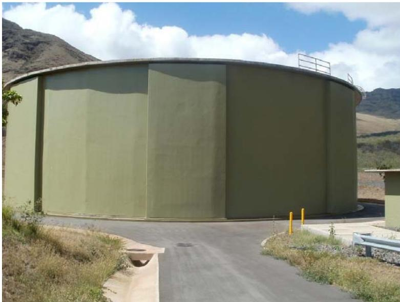
**Reservoir Construction.** *The newly constructed Nanakuli 242 reservoir adds two million gallons of potable water storage capacity for the Leeward water system .*
