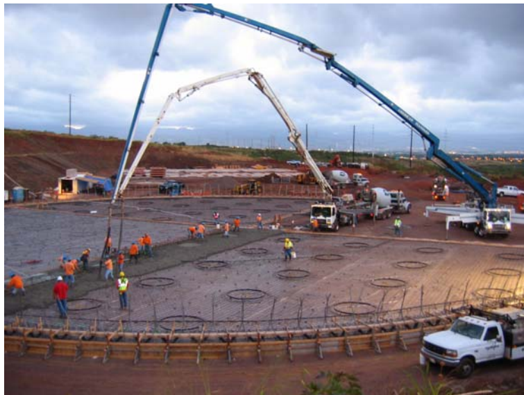
Reservoir Construction. Crews work on the foundation of the new Honouliuli 228 Reservoir No. 3.
