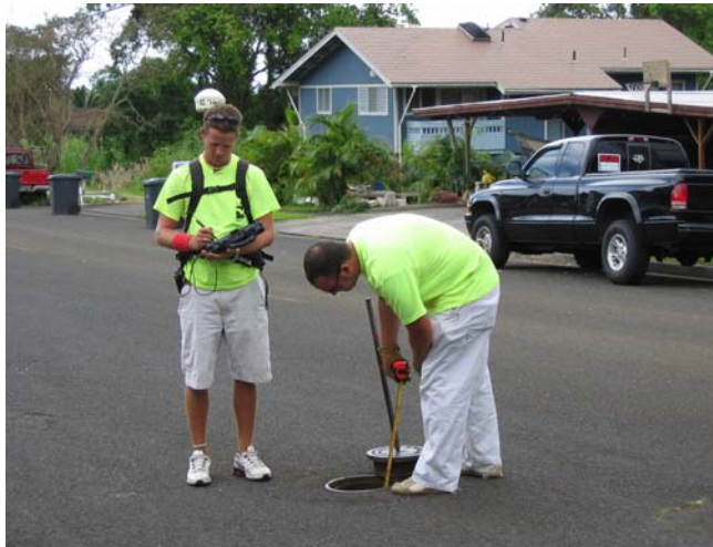
Asset Management. Contractor's help map BWS assets using Global Positioning System technology.
