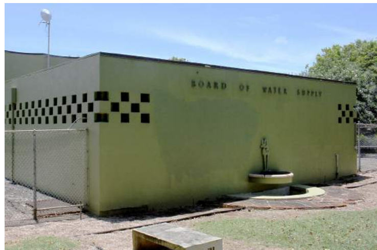
Wai'ālae Iki Booster - To secure two major facilities away from a tsunami zone, BWS will abandon an existing booster pump and relocate another booster up a hill to the Wai'ālae Iki Reservoir site.
