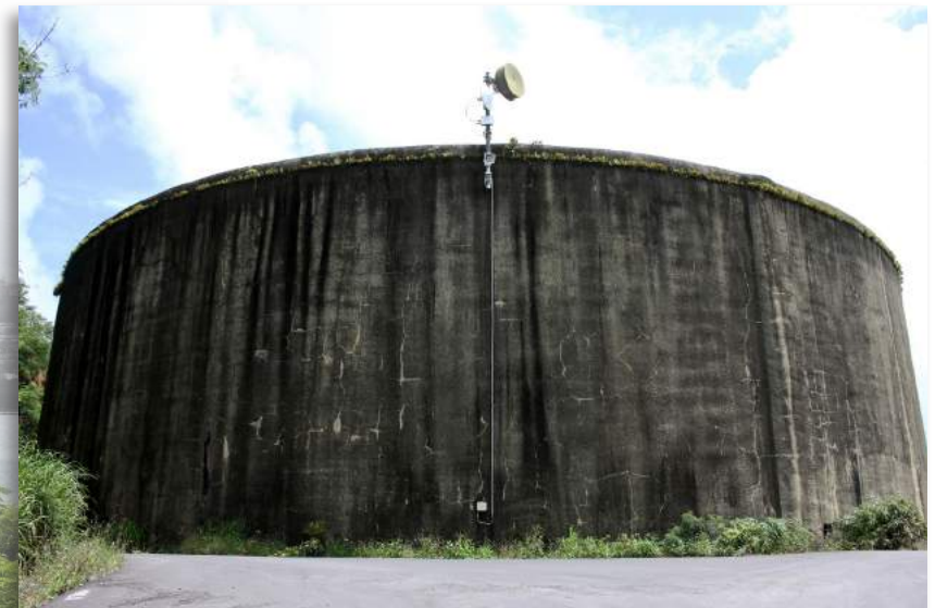
Kapa'a Reservoir Improvements - Leaks have been discovered in the wall of this reservoir, built in 1957. To simplify installation and provide additional options for water system operation, this 2-million gallon reservoir will be replaced with two, 1-million gallon reservoirs.
