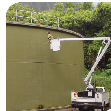
Inspector conducting an assessment of a BWS reservoir
